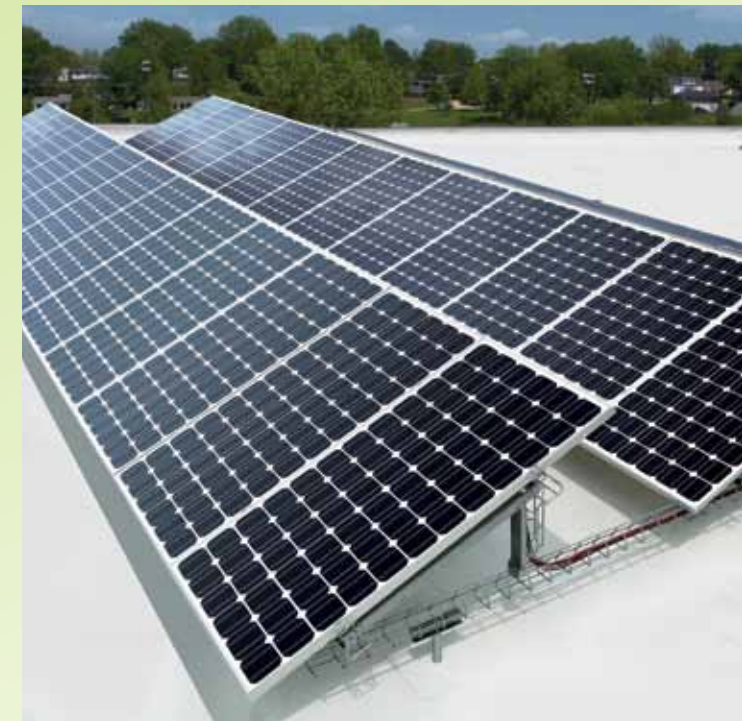
Stanchion mounted Delta Strut on membrane roof
