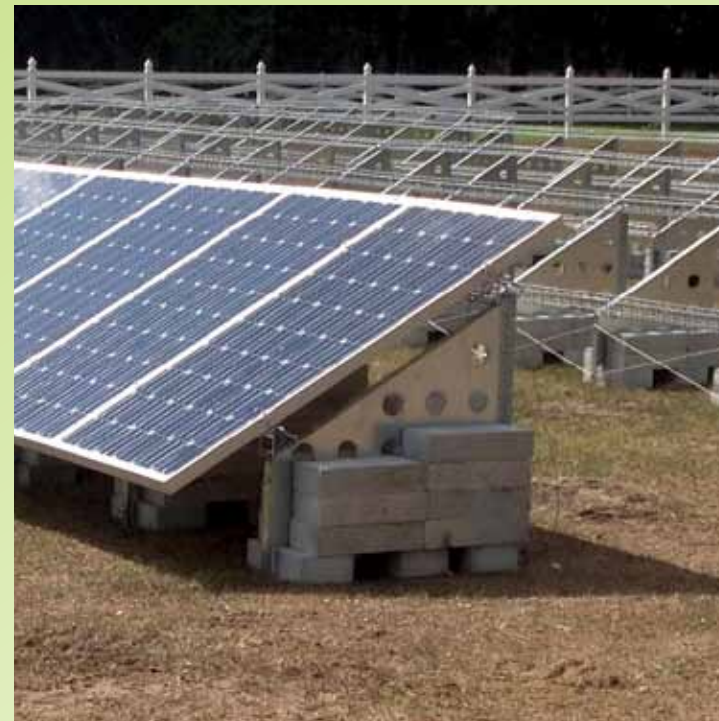
PV panel supports with ballast on sandy soil
