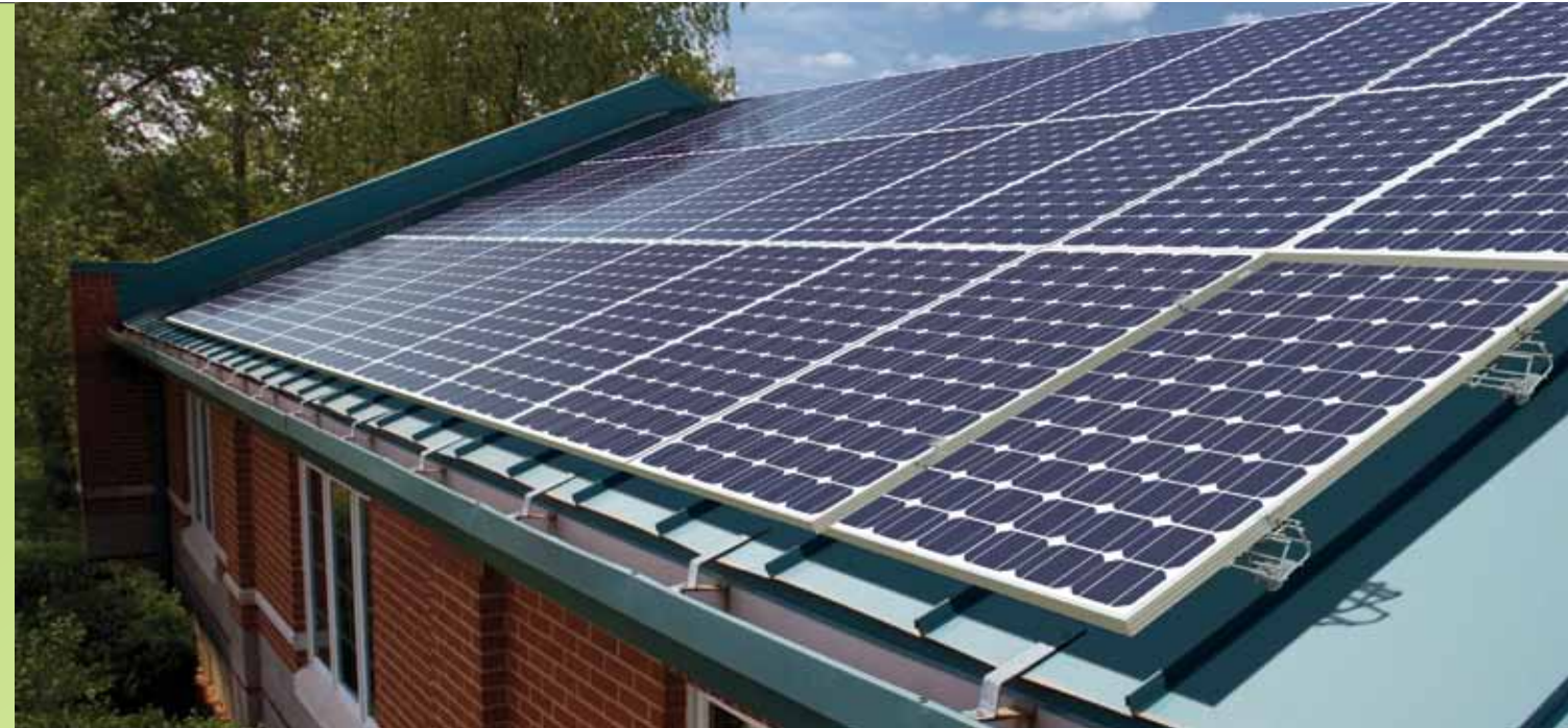
Delta Strut attached to standing seam roof
